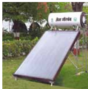
Hot plate collector
