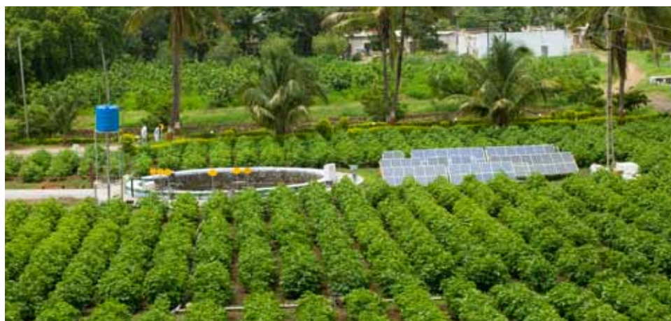
Installation of solar pumps for Drip Irrigation Systems
