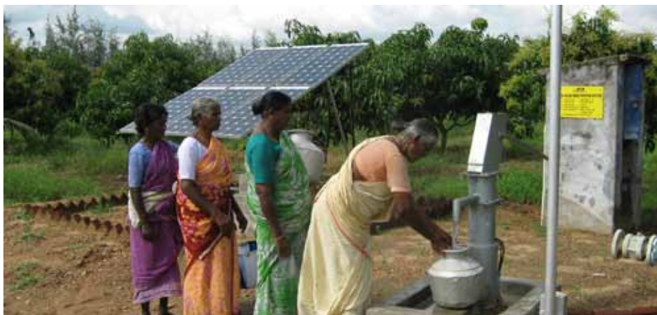
Installation of Jain Hand+Solar Pump
