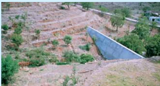
Masonry retaining wall in Neem Valley does not store even a single litre
