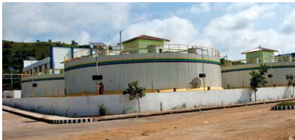
View of Biogas power plant
