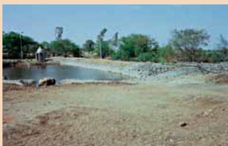
Percolation tank filled with water
