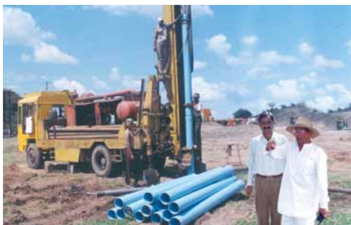
Bhau and P. A. Patil with boring rig
