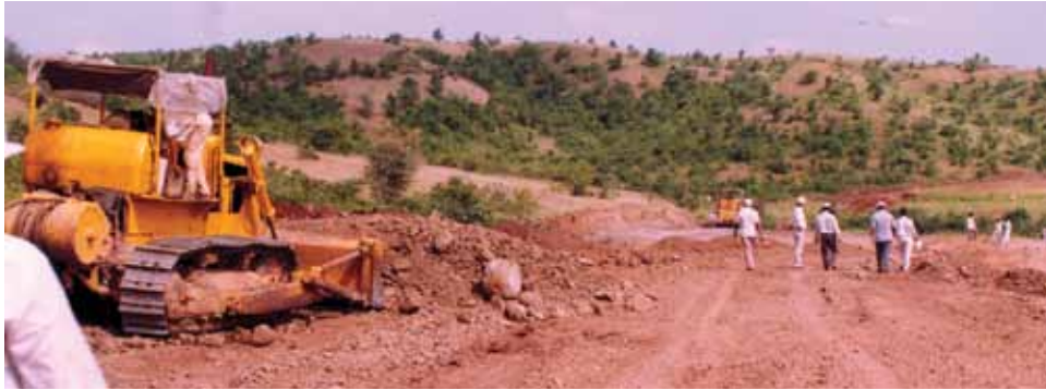
Land levelling with a caterpillar bulldozer
