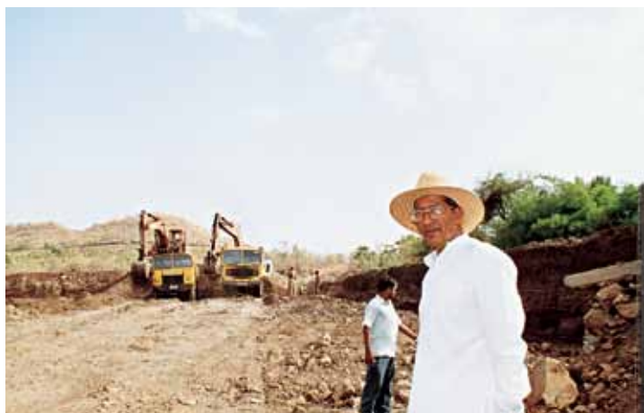
Bhau smiling at site : Rebuilding of percolation tank, Sindhu.
