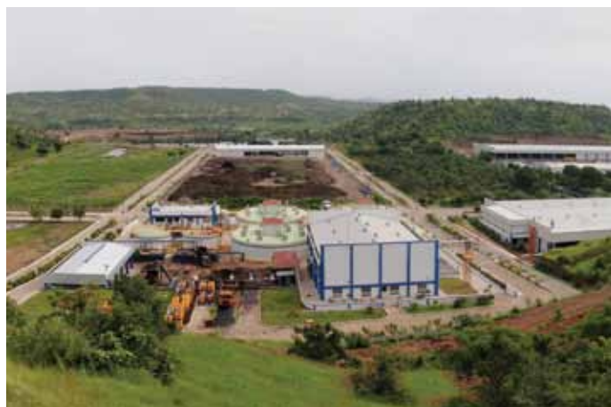
Bird’s eye view of Green Energy Park
