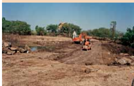
Construction of earthen bund
