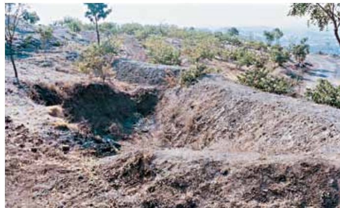
Earthen gully plug
