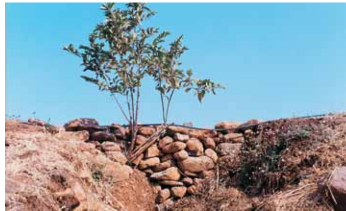
Dry rubble gully plug
