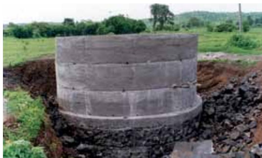
Hybrid construction with UCR and RCC rings in a dug well
