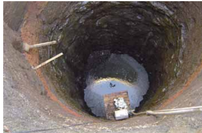
Artificial recharging of a dug well
