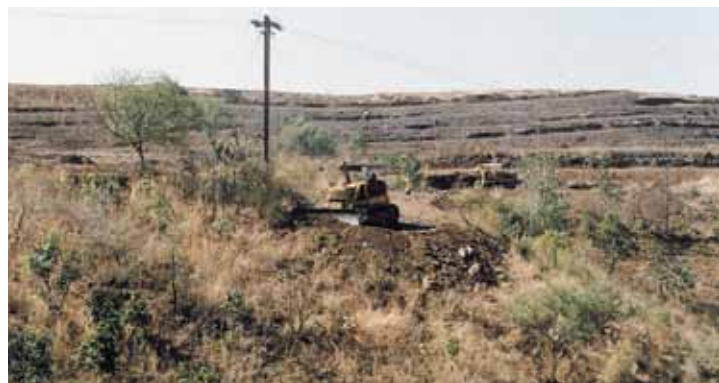
Bench terracing work in progress with a bulldozer
