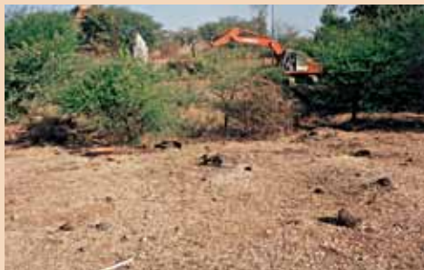
Site clearance work in progress
