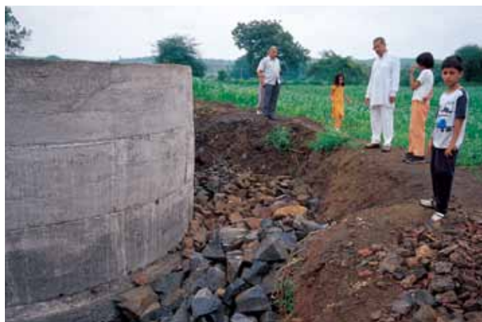
The future generation inquisitive about filter bed for recharging of dug well. Technical advisor Shri. V. R. Barve looks on.
