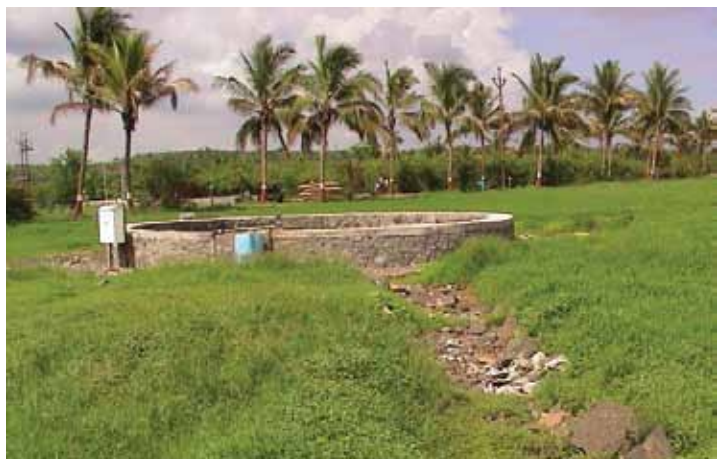
Dug well with open collection trench and artificial recharge arrangement
