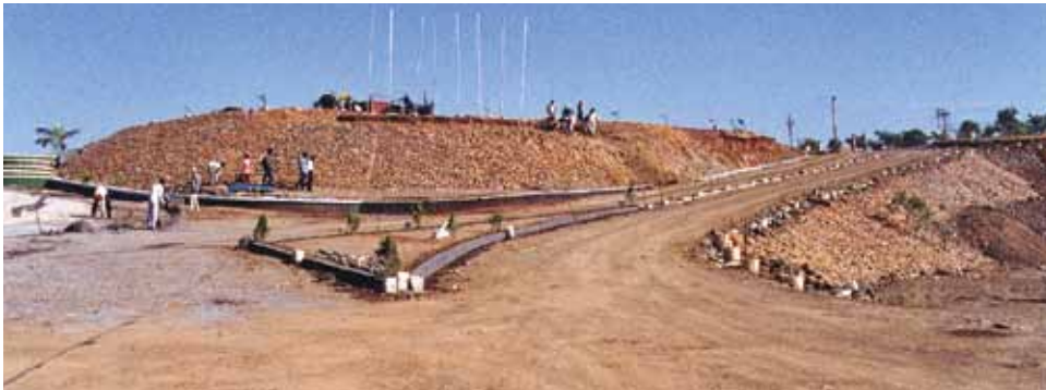
Stone pitching on steep slopes
