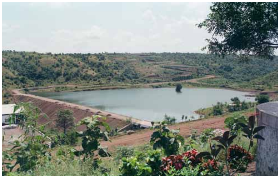
Jain Sagar Percolation Tank
