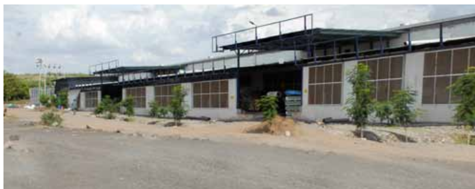
Solar Water Heating: Production Unit
