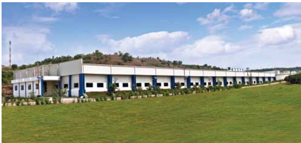
View of solar photovoltaic module manufacturing plant
